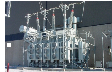
A 345 kV 360 MVA transformer used for high voltage power distribution
